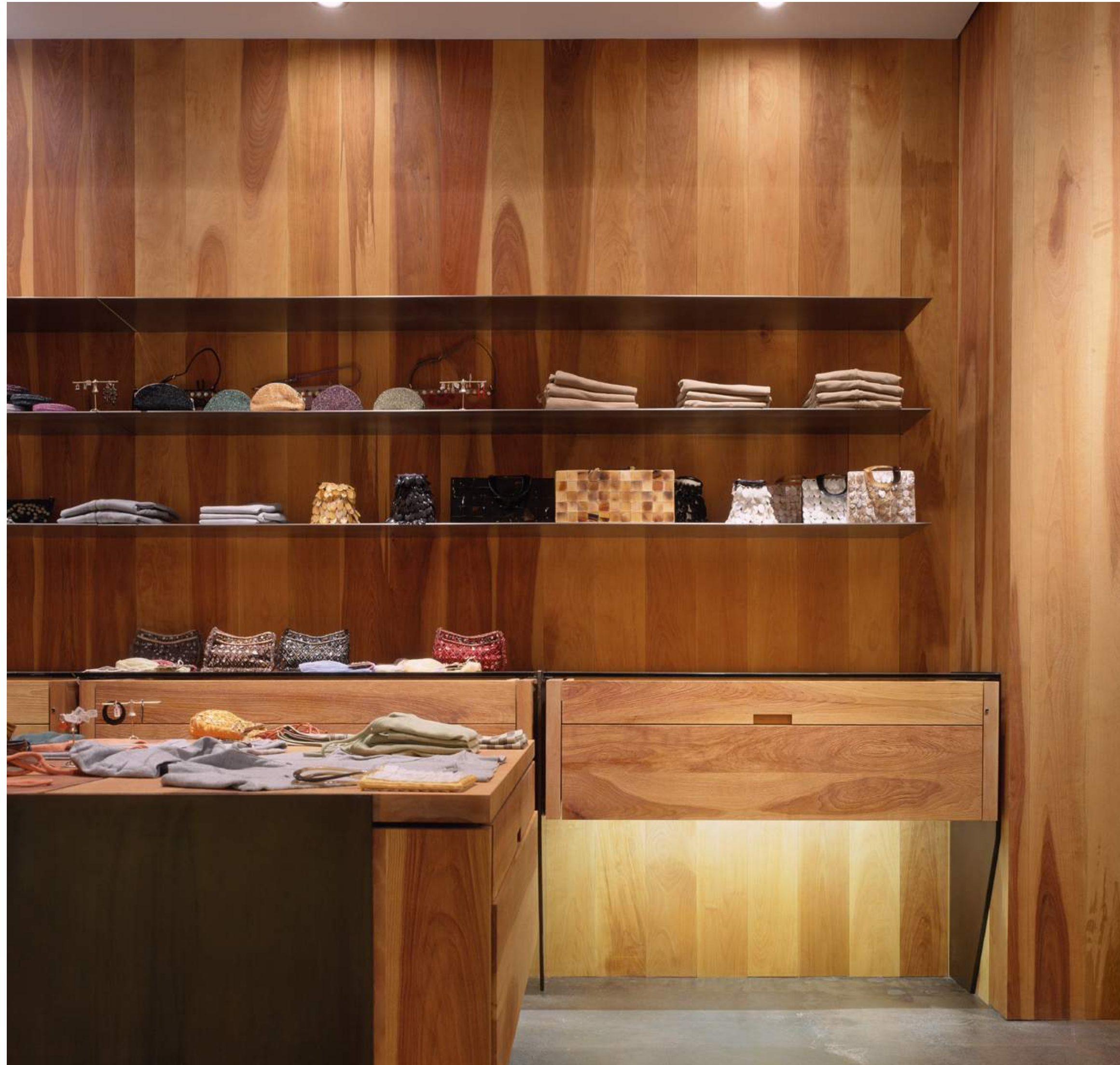
Sandblasted birch wall paneling and casework, Chan Luu
