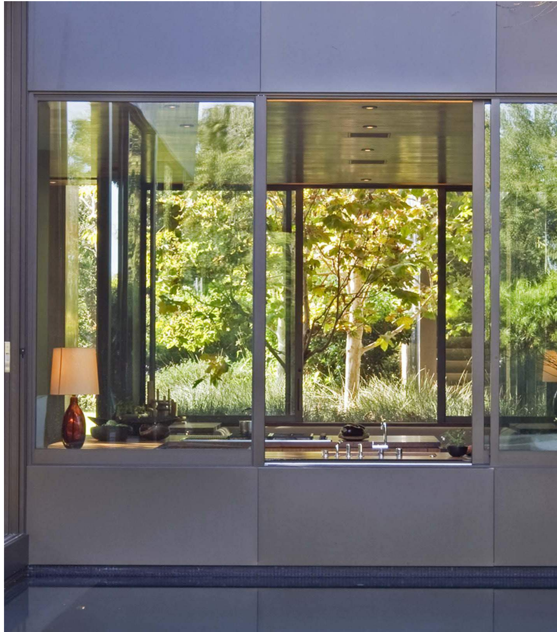
Bronze and anodized aluminum panels, Vienna Way
